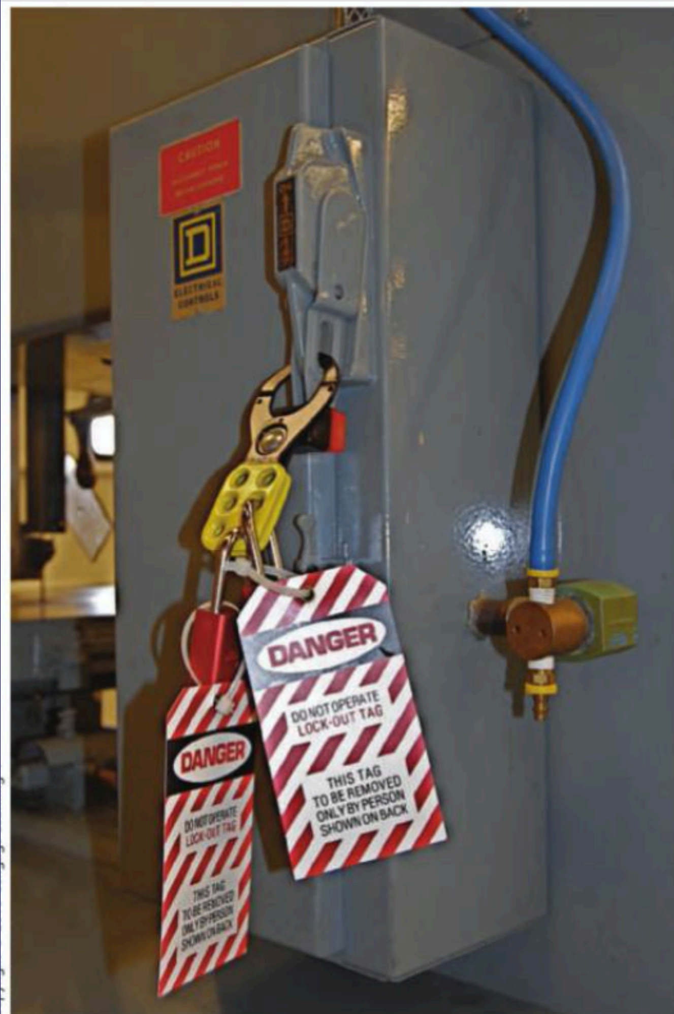
FIGURE 2.1.16 A lockout hasp allows several different people to lock out or tag out a piece of equipment. This machine has been locked out by two different people.
